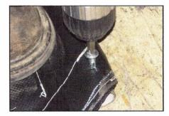
Place the plastic end caps into each end of the anchor pipe. Fasten each end of tarp to the anchor pipe with the 1/4" tek screws supplied.
