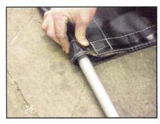
Unfold and straighten tarp. Insert the anchor pipe into 4" pocket and slide thru to other end. Cut both ends flush with edge of tarp.
