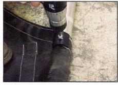
Fasten tarp to roll pipe at rear with "U" clamp and 1/4" tek screws provided. Install "U" clamps one on every seam apart down the length of tarp.
