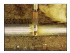
Roll pipe and anchor pipe is supplied in 20' joints. Assemble and weld joints. Insert gudgeon in end of roll pipe and weld as shown.
